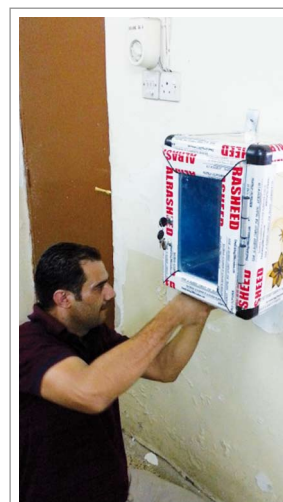
The staff is fixing an enclosure for Face ID 2 to avoid vandalism
