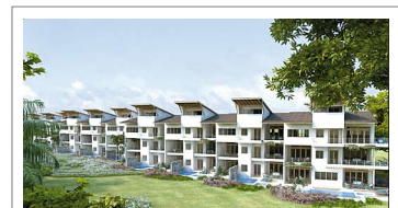
View of part of the residential buildings in the community
